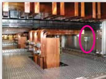
Examples of Arc-Flash Relay light sensor installation in switchgear.
